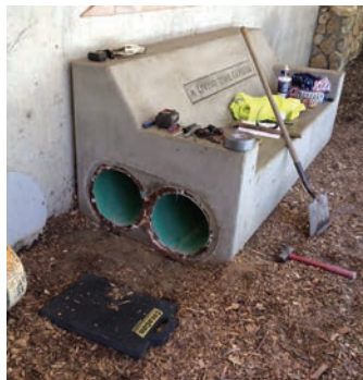
The capsules are 12" diameter PVC pipes.
